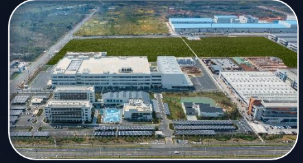
Guangde Factory (Phase III), China
