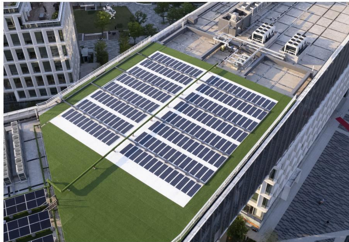
Rooftop terrace, China Tower Corporation Limited
